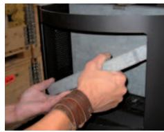
22. Insert the horizontal stone at an angle and rotate it gently into place.
