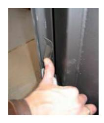
9. When the side stone is in place, install a spring (6 provided) roughly at the middle of the stone.
