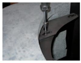
32. When the top panel is in position, tighten these screws so that it cannot move.
