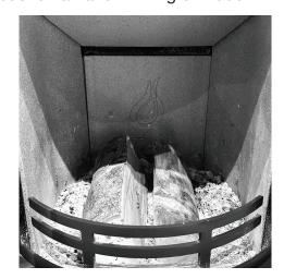
Ensure when refueling that the wood is not too close, it will cause poorer combustion, less heat out-put and lower efficiency.
