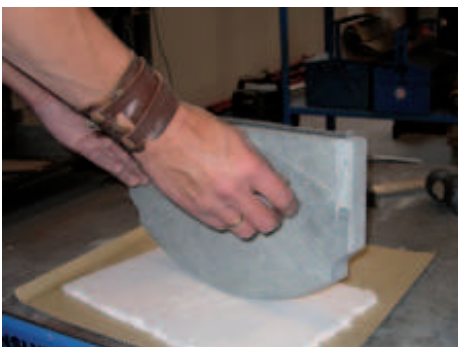
21. Protect the stones during installation.
