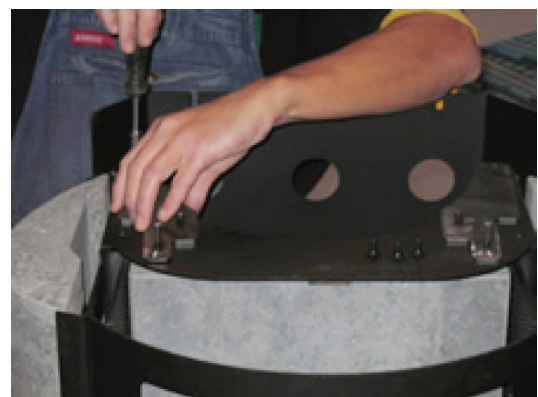
25. Attach the two brackets supplied.
